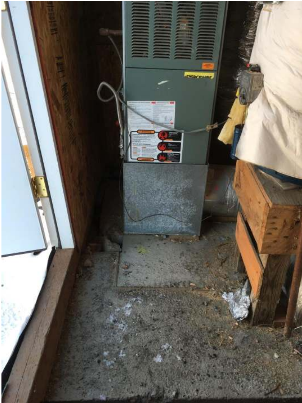
Photograph #6: Mechanical equipment on concrete pads in the addition.
