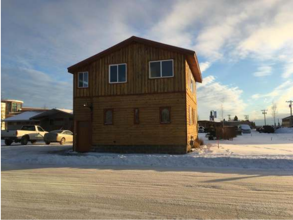
Photograph #1: Front (northwest side) of the building at 509 Overland Avenue.
