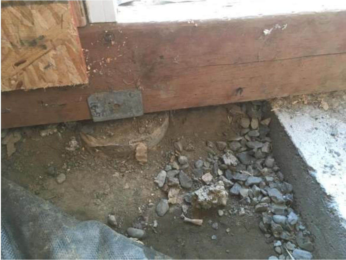
Photograph #2: Bottom of exterior wall of addition. Note lack of a continuous footing under the wall.
