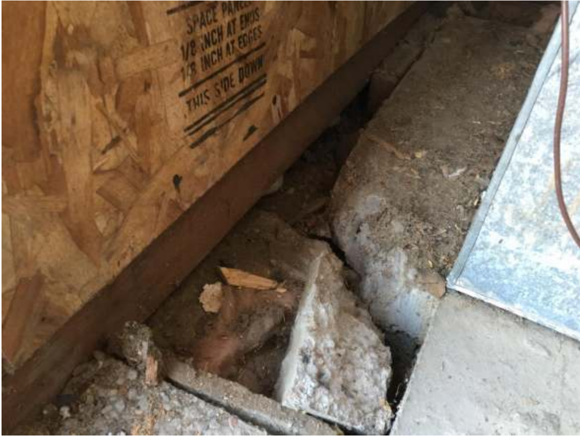
Photograph #3: Bottom of exterior wall of addition. Note lack of continuous footing under the wall.
