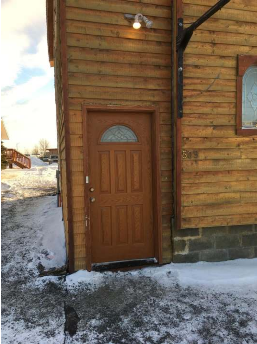
Photograph #4: Front (northwest) wall of addition.
