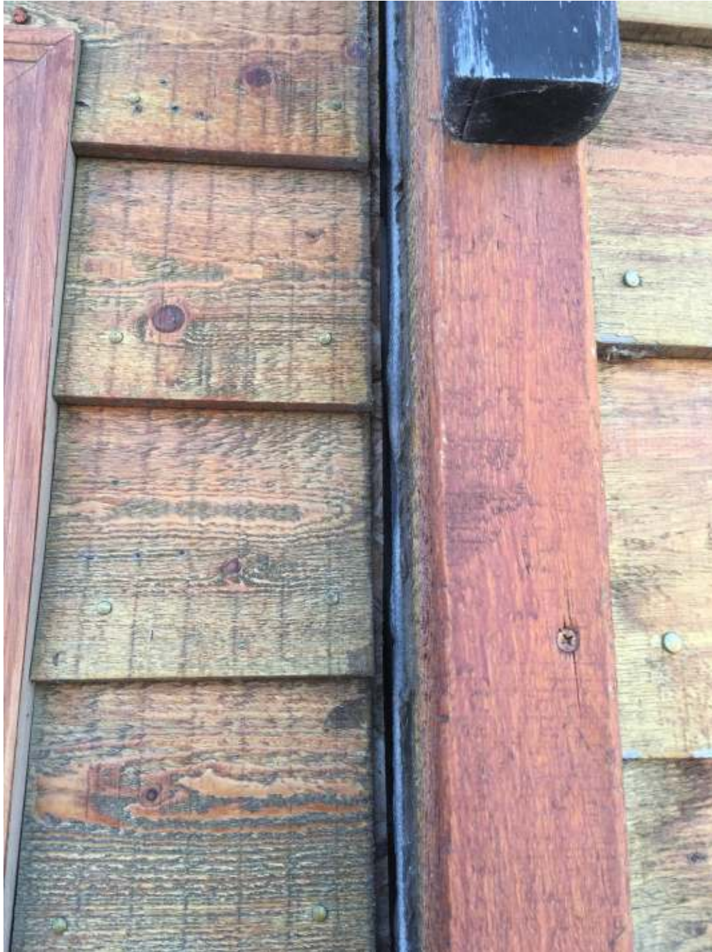
Photograph #5: Approximate 1/2" wide gap between addition (left) and main portion of the building (right) on front wall.
