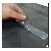
c) Press section firmly back into place. Repeat this process along the length of the mat, then repeat for other side.
