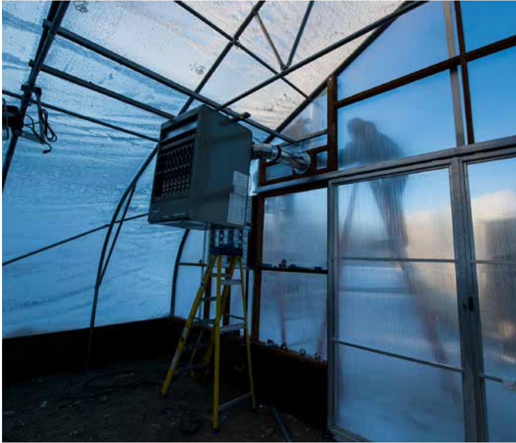
Clayton Simpson and Tyler Crane with Crane Plumbing and Heating work in December to install a heater for one of the Tribe's two greenhouses.
